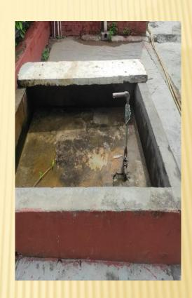
Bore well /Open well recharge: In our College Bore well and open well recharge are methods used to replenish groundwater levels by allowing rainwater to percolate into underground aquifers. Here's a brief explanation of these processes:
